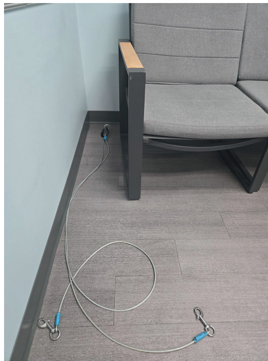
■ Fig. 1.3. These ringbolts are screwed directly into cement flooring. Metal tethers can then be connected to patient collar or harness for additional staff safety.
